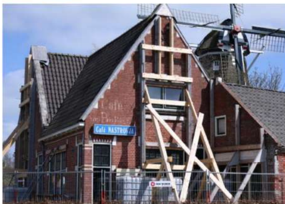
A condemned and shored-up cafe in Zeerijp. Photo: Graham Dockery
